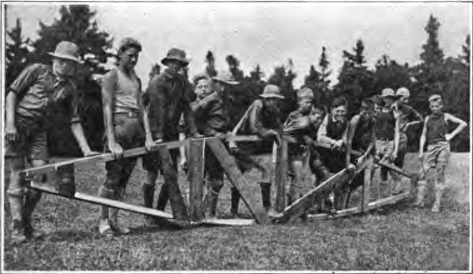
ONE SIDE OF THE FIRST SPAN (16 FOOT) COMPLETE
